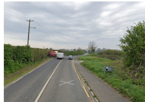
7. Existing road connecting Coill Dubh and Cooleragh (L1019)
