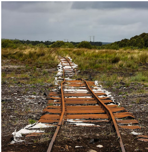
Existing train tracks through bog lands
