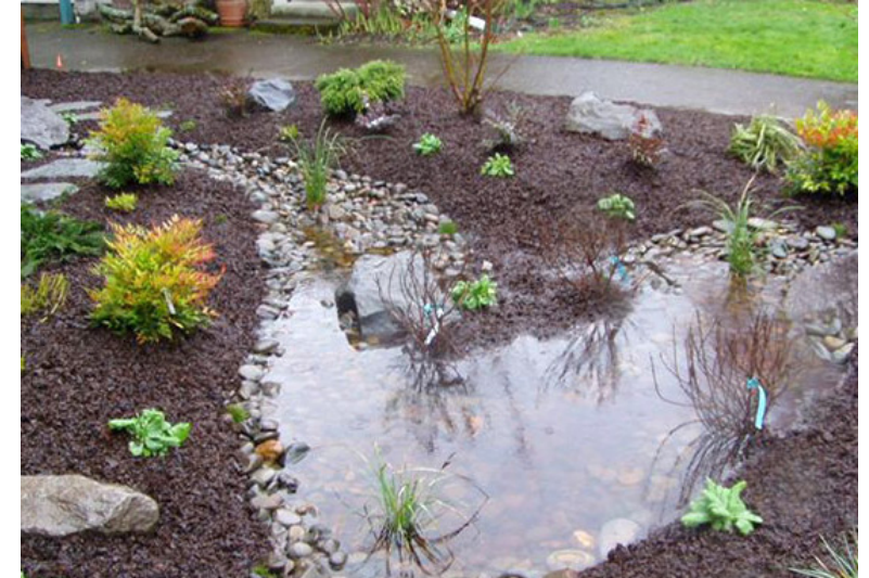
Rain Garden - Sustainable Drainage Systems (SuDS)
